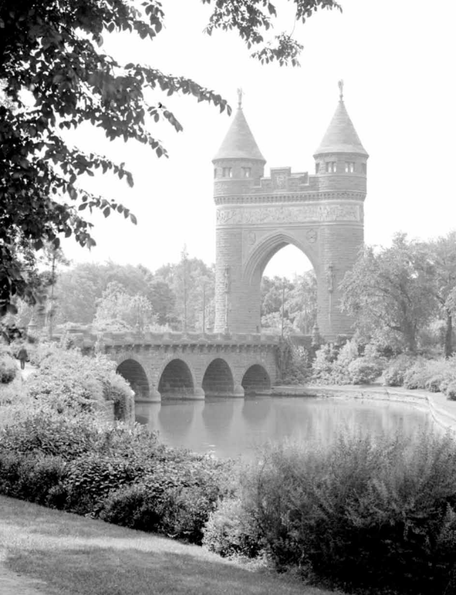
The Ford Street bridge, with its graceful stone arches, was completed across the Park River in 1850. Bushnell Park was completed ten years later, and the Memorial Arch was added in 1886. In the 1940's, the river was diverted to an underground conduit, and the bridge was buried in place. The Bushnell Park Restoration and Extension Plan would uncover the bridge and restore flowing water through its arches.
