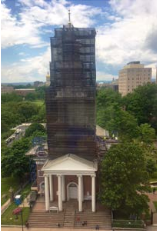
2017 restoration of the Center Church steeple
